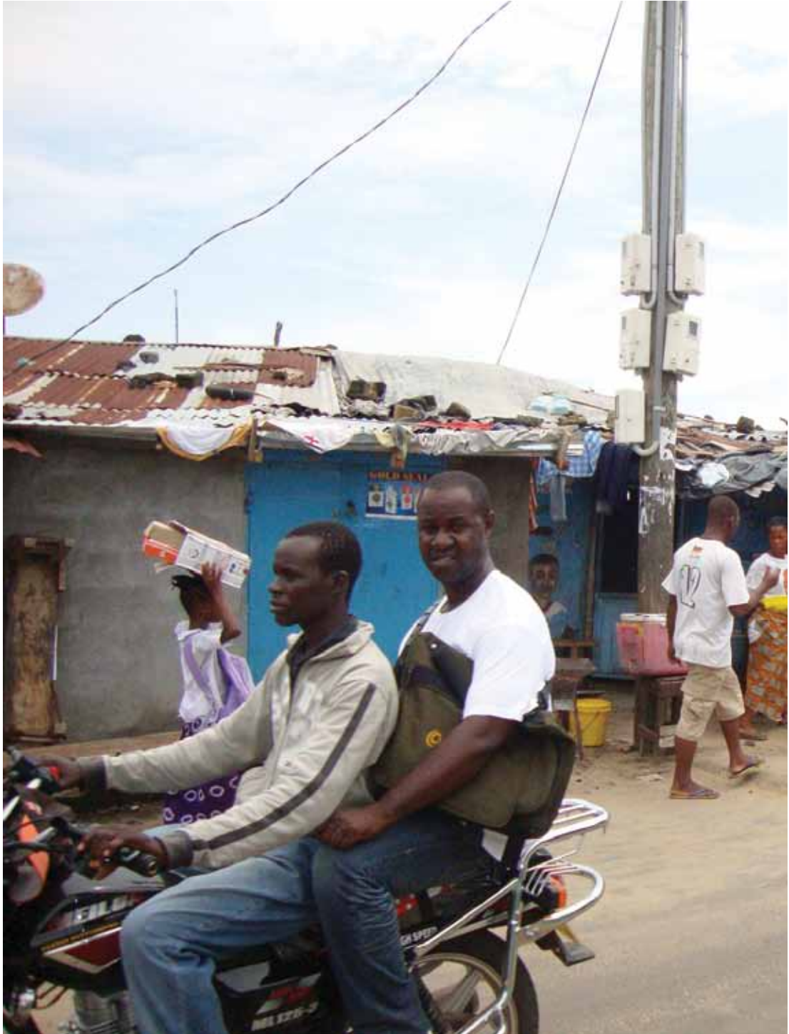
Neighborhoods such as these have benefitted from the recent efforts to extend the electricity grid. West Point, Monrovia.
